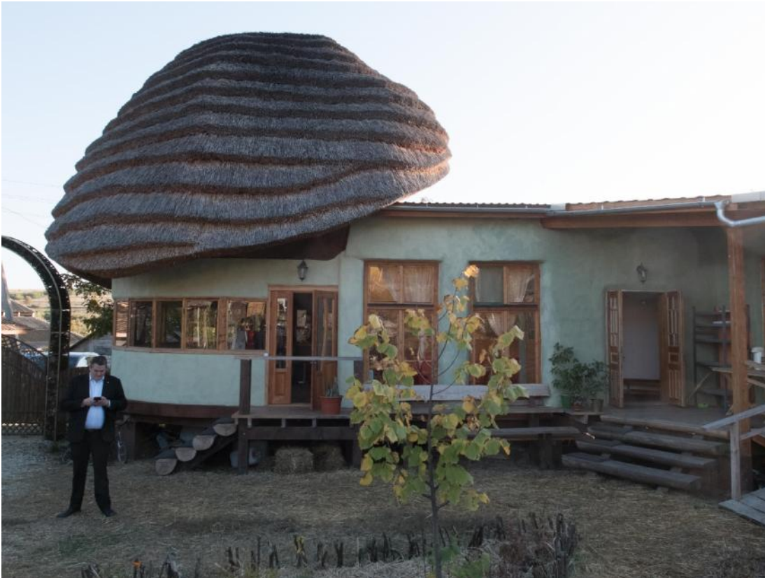
Photo of the Eco village green building with its straw roof
